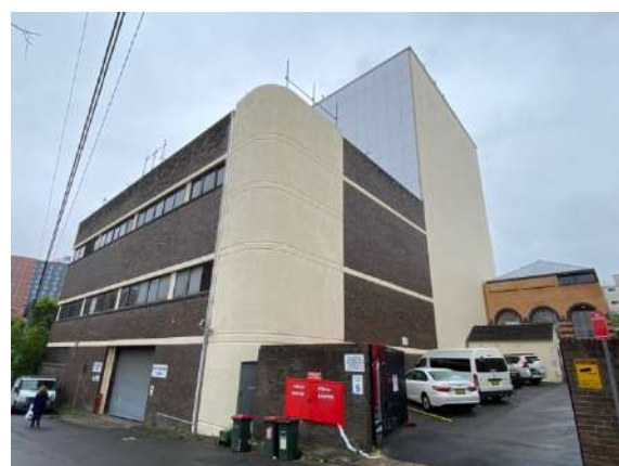
Figure 5: Photo taken from Turner Street showing the 1974 telephone exchange building and the neighbouring St Vincents church building to the right rear.
