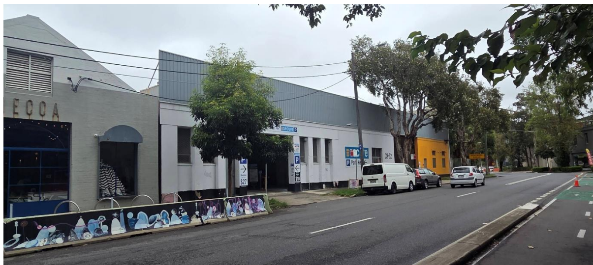
Figure 6: Western adjoining site at 28-32 Bourke Road
