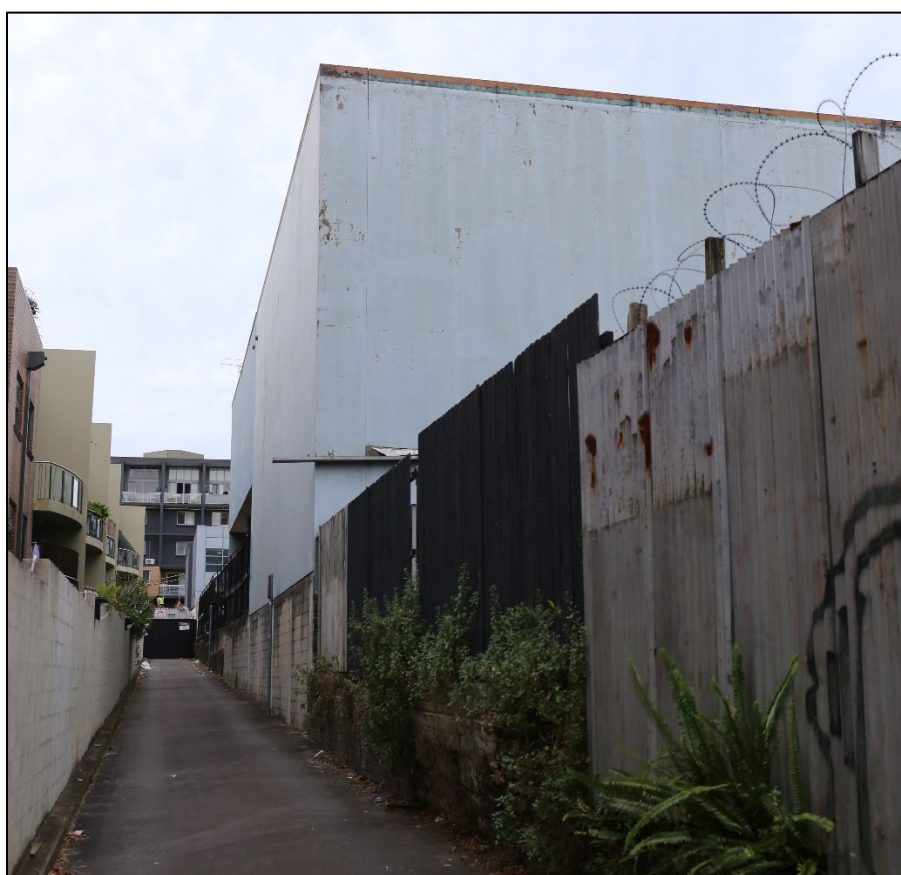
Figure 6: View from Cornwallis Lane looking north with site located on right of lane
