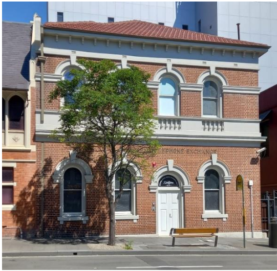
Figure 2: 117A Redfern Street, Redfern. Source: https://www.facebook.com
